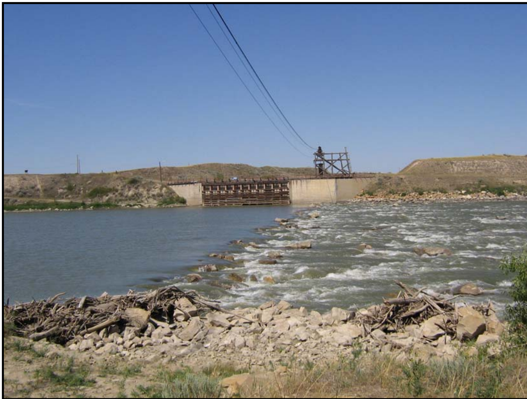
Figure A.2.4 - Dam Crest 25 August 2008.
