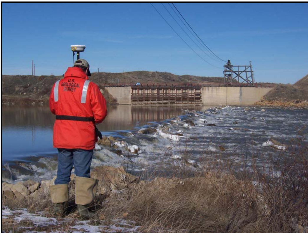
Figure A.2.3 - Dam Crest 2 November 2006.
