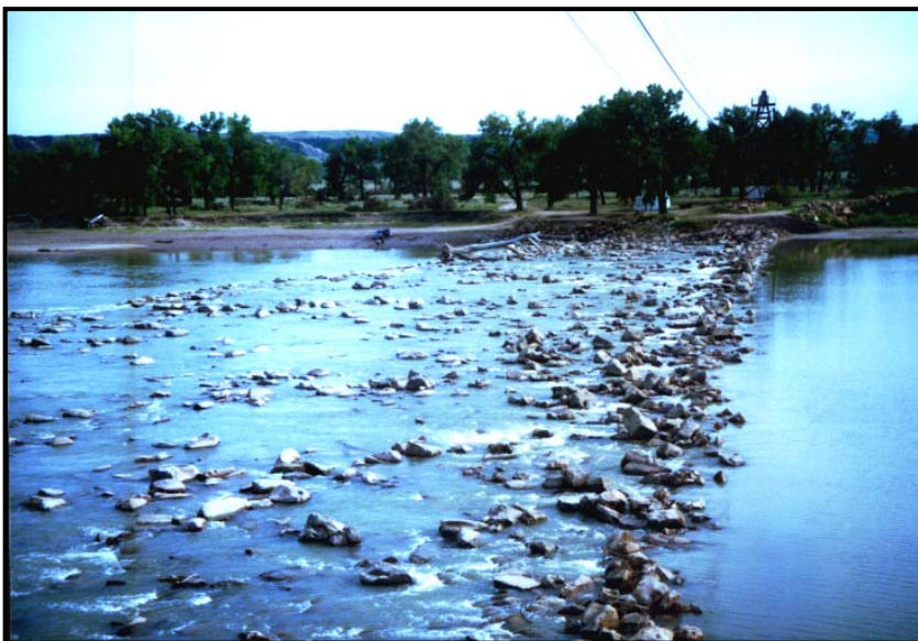
Figure A.2.1 - Intake Diversion Dam at Low Flow.
